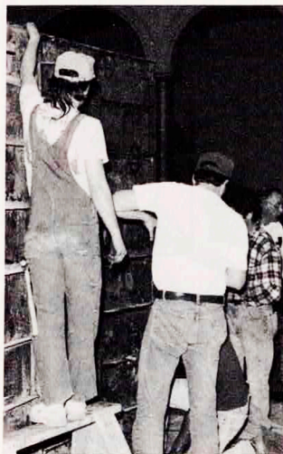
Union apprentices from the Joint Carpentry Apprenticeship Committee of Washington, D.C. and Vicinity set in place a Steel-Flex form (provided by the Symons Corporation, Des Plaines, Ill.), as part of the "Moving Circles—Art at Work"
