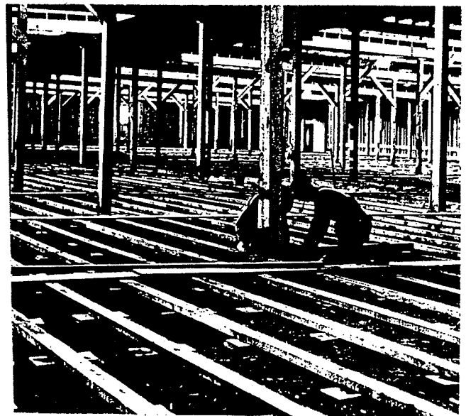
Exposition hall being prepared to house Japanese Americans, 1942
